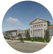
Walnut Hills Renovation and Expansion Summer 2022
