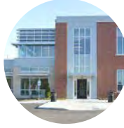
Price Hill Renovation and Expansion
