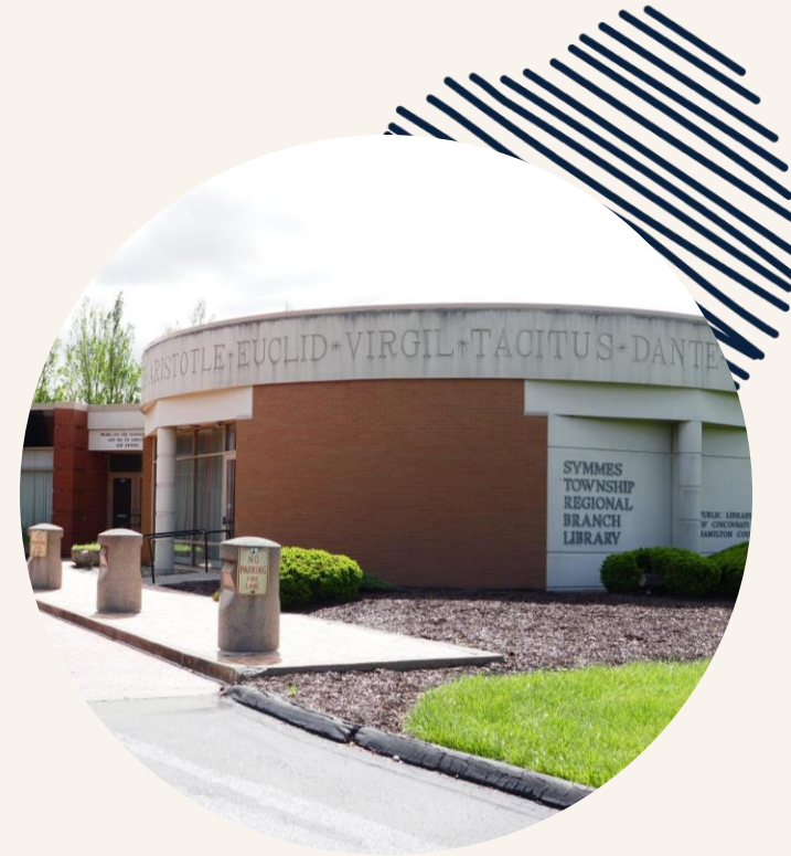
Symmes Township Renovation Expansion
