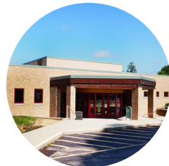
Delhi Township Renovation or Replacement
