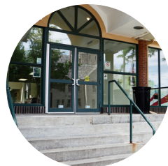
Oakley Maintenance and Interior Updates
