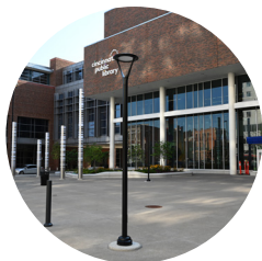
Main Library Maintenance – Chillers and Cooling Towers Replacement
