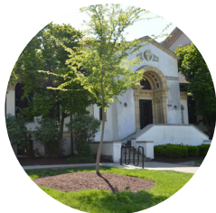
Avondale Maintenance and Interior Updates
