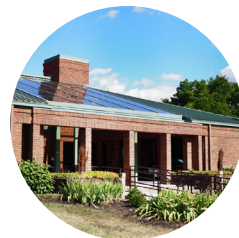
Mariemont Maintenance and Interior Updates
